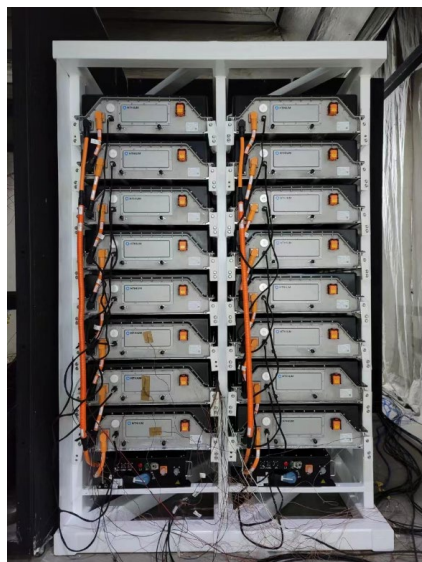
Figure 4. BESS Rack
